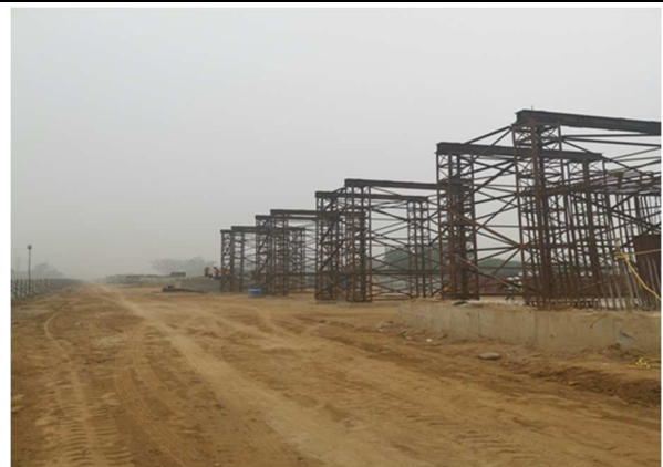
FIG 7 – LAUNCHING GIRDER STAGING AT ELEVATED STRUCTURE
