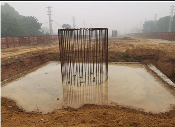
FIG 6 – PIER WORK IN PROGRESS
